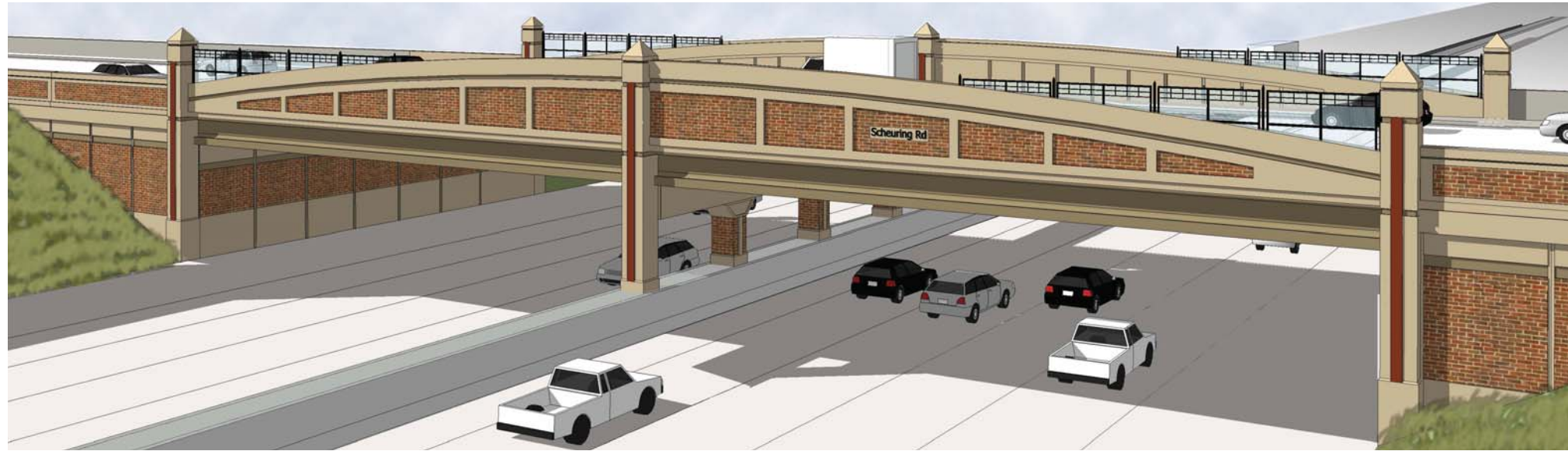
Arched Parapet, local street over US 41 at Scheuring and Lineville Rd
